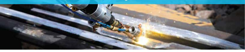
Railroads report that traditional repairs to frogs and diamond inserts often only last weeks to a few months before requiring additional maintenance. These specialty track components are manufactured out of cast austenitic high manganese steel known for its excellent work hardening characteristics and high toughness. However, this material creates a unique challenge to repair or refurbish in the field as it cannot exceed 500 degrees Fahrenheit.
